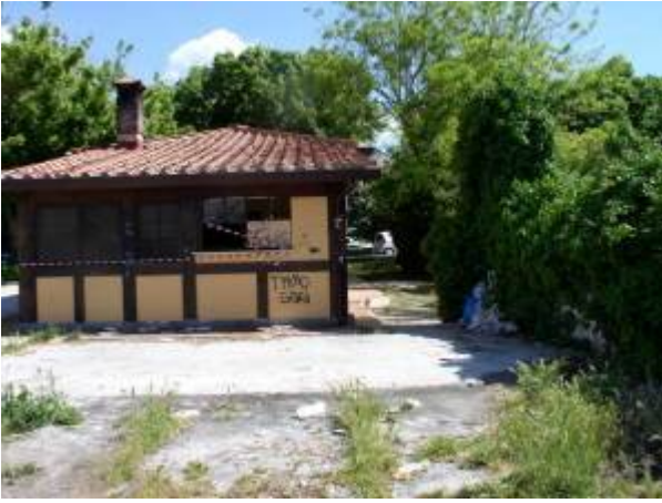
Grottaferrata, area abbandonata
